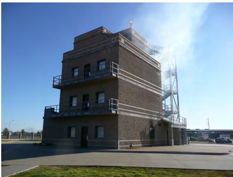
Figure 1. Cinder-block tower during a training exercise.
